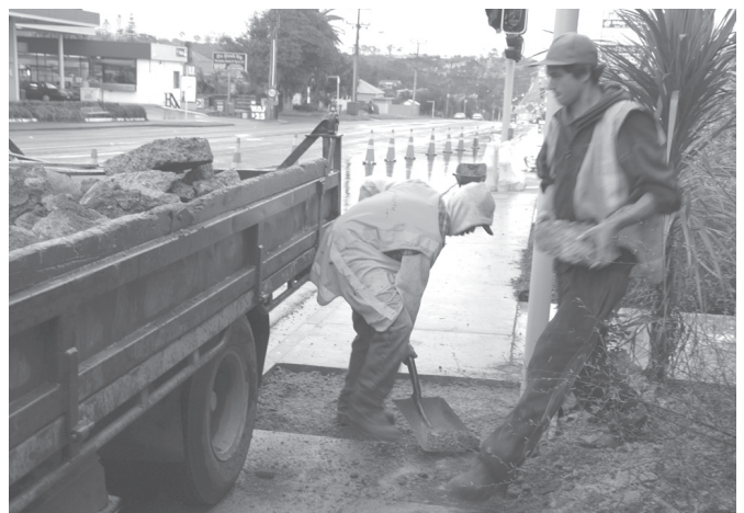
Footpath improvements, Glen Eden
