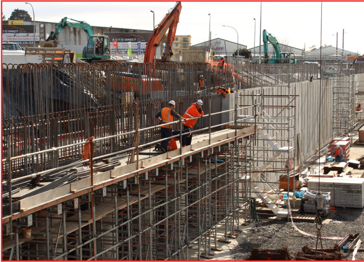
Busway bridge abutment
