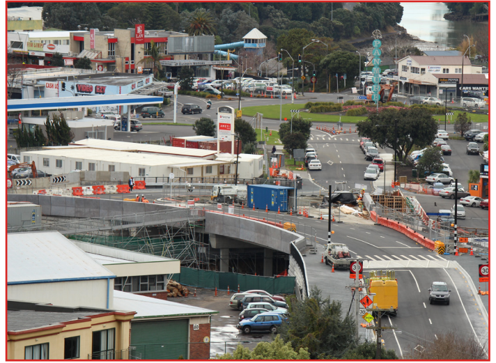
Mountain Rd bridge open
