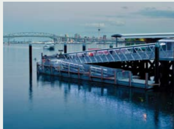
Birkenhead Wharf, refurbished, was re-opened in June 2012.
