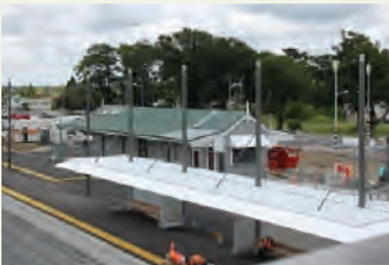
Looking towards the Papakura station ticket office
