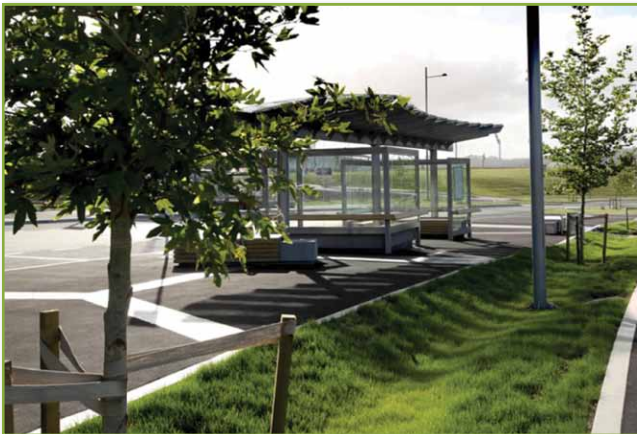
Figure 6.5-1 Low impact design feature – grass swale at the ALP Source: Anguillid Consulting Engineers and Scientists Ltd
