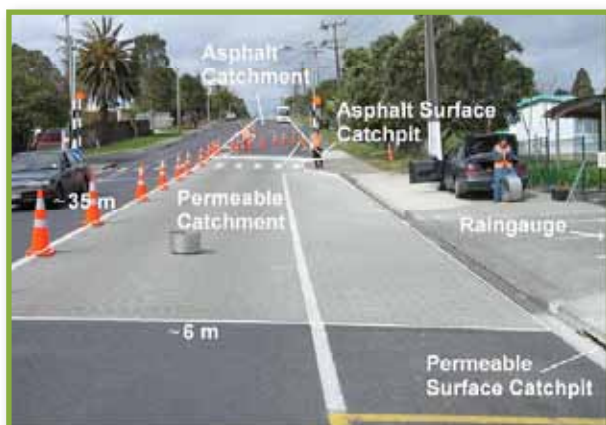
Figure 5.4-7 Permeable pavement section on Birkdale Road
