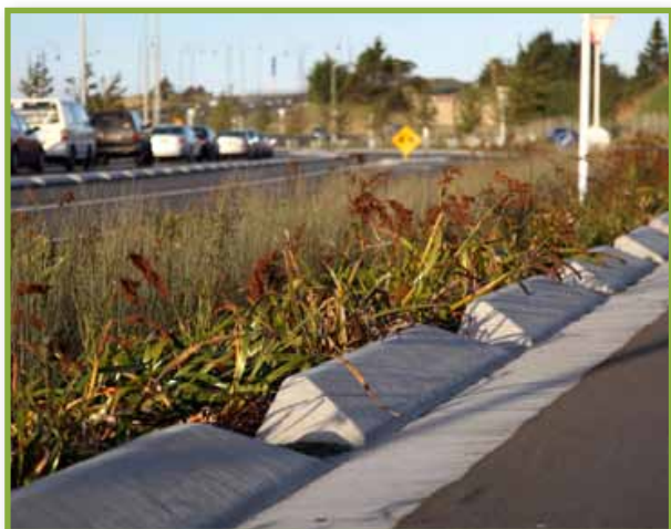
Figure 5.4-1 Rain garden – Albany Lakes Precinct Source: Internet
