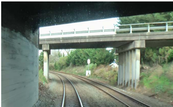
Bridge 3 (Northbound Off Ramp) Travelling South
