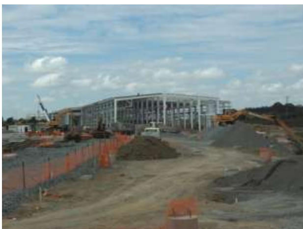
Figure 2: View north - first trackwork going in
