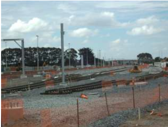
Figure 3: Overall site view to south
