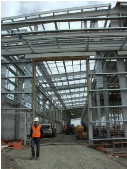
Figure 4: First roof sheeting going on
