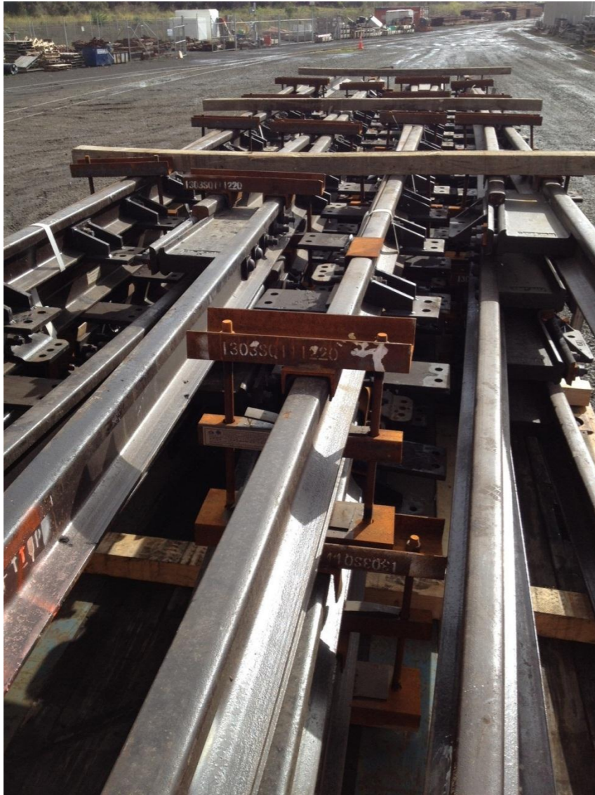
6 kms of track delivered
