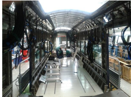
Fig 2: The inside of the Trailer Car, structural floor in place and being wired
