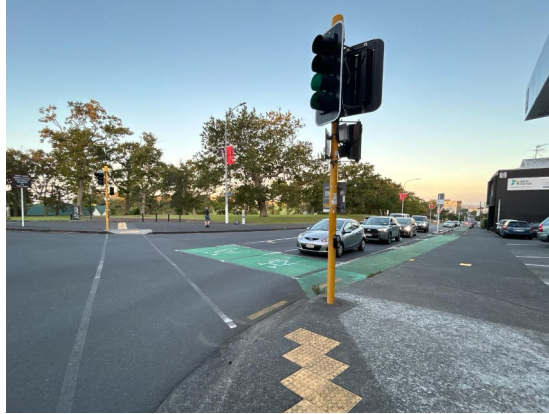
Figure 23: Physical separators change to hatch marking buffer to allow people cycling to move across to the right-turn ASB on Carlton Gore Road – Park Road intersection
