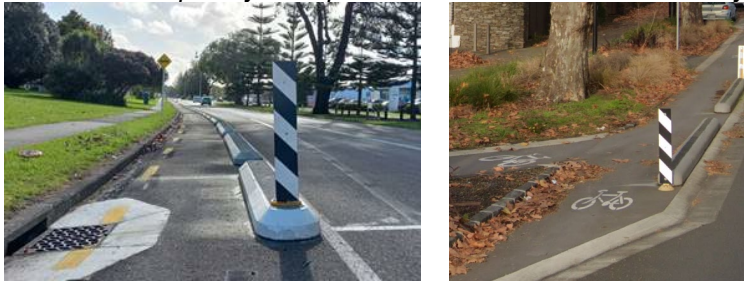
Figure 13: Bridge Marker Post Location
