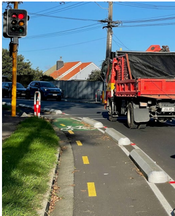
Western approach to head of T-intersection Mount Albert Road and Frost Road
