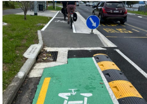
Figure 19: Example of catch pits at raised safety platform (Source: Auckland Transport)
