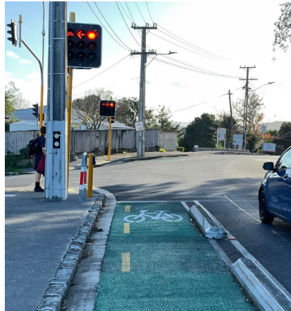
Figure 26: Eastern approach shows left turn cycle traffic light control with separators up to the stop line on Mount Albert Rd and Frost Rd (Source: Auckland Transport)
