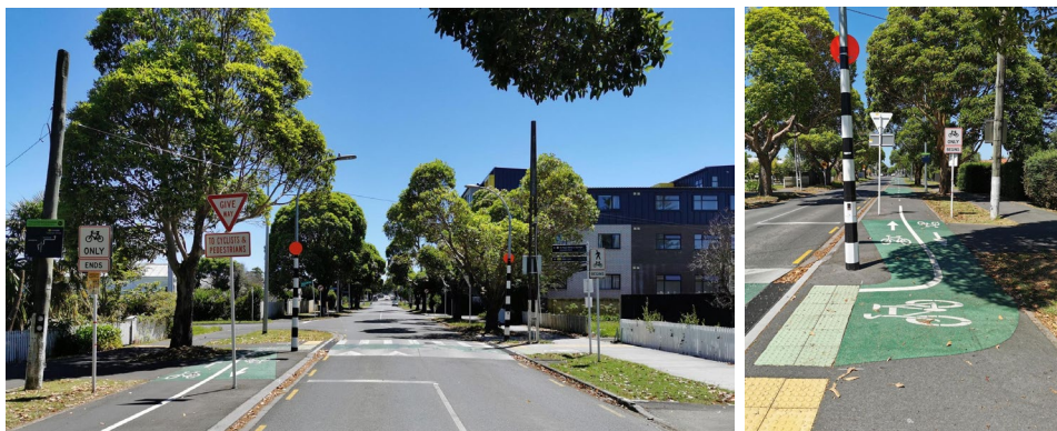
Figure 17: Bend/turning tracking and signage location need to be accounted on the design. Location: St Georges Rd, Avondale (Source: Auckland Transport)
