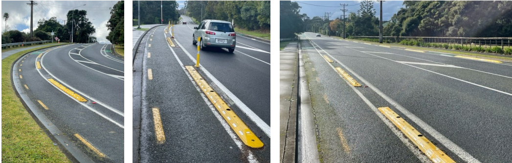
Figure 8: Upper Harbour drive Example of use of rubber Flexible Traffic Separator (Source: Auckland Transport)
