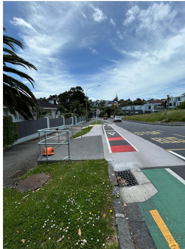
Temporary bus stop at Ngapi Rd cycleway
