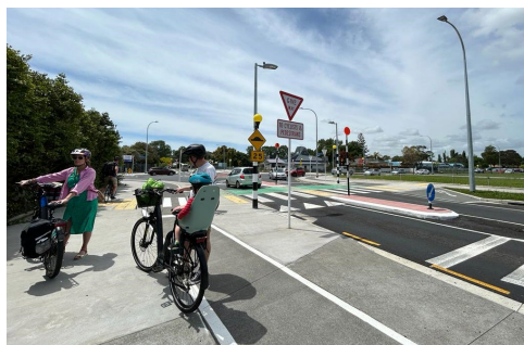
Figure 20: Separated cycleway on the single lane roundabout on Taniwha St – Elstree Ave (Source: Auckland Transport)
