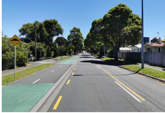
Figure 10: Raised lane separator using mountable kerb on St. Georges Road, Avondale
