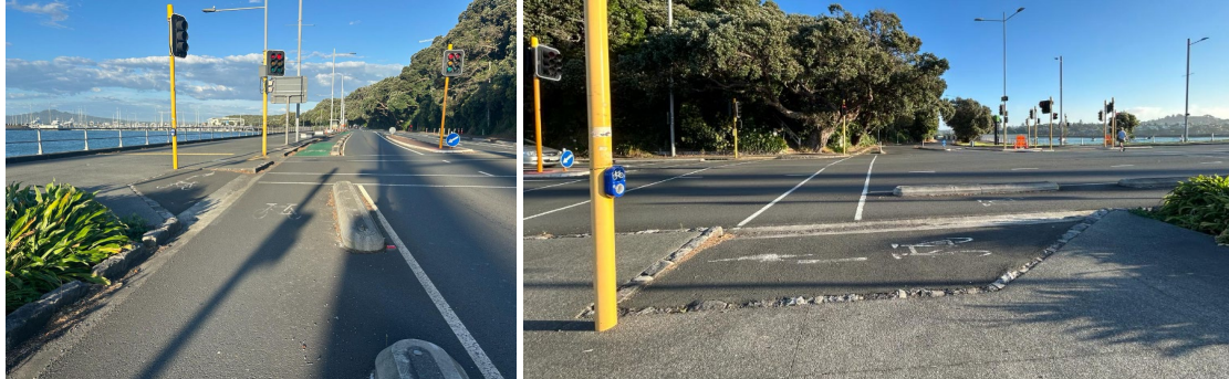
Figure 24: Jug handles provide waiting space for people cycling who want to turn right at the T-intersection of Tamaki Dr and Ngapipi Rd (Source: Auckland Transport)
