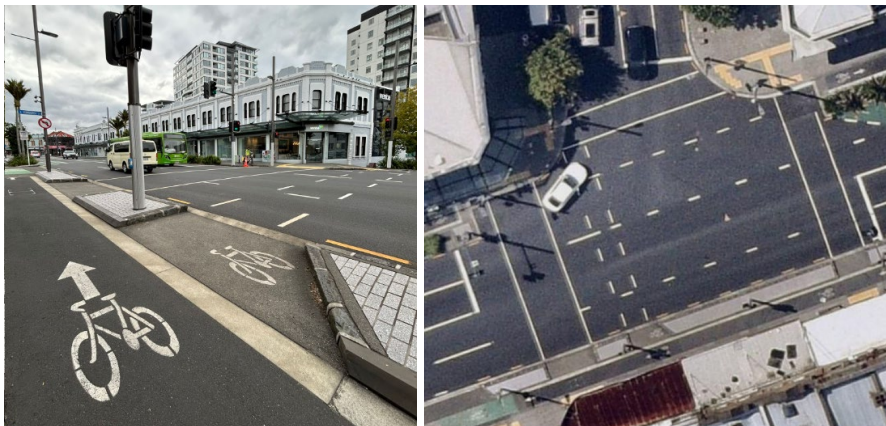
Figure 25: Separator gap: waiting space for people cycling to turn right at T-intersection of Karangahape Rd and Howe St (Source: Auckland Transport)
