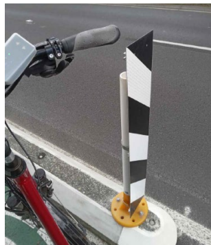
Figure 12: Bridge Marker Post (Source: Auckland Transport)
