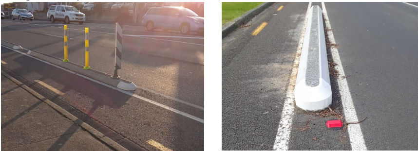
Figure 9: Painted concrete cycle separator (Source: Auckland Transport)
