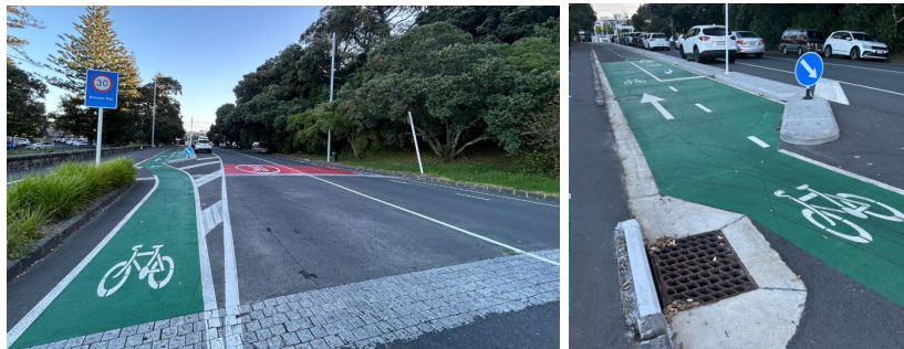
Figure 37: Shared Path, one-way directional on-road cycle lane, and separated two-way directional cycleway connection on Tamaki Dr (Source: Auckland Transport)
