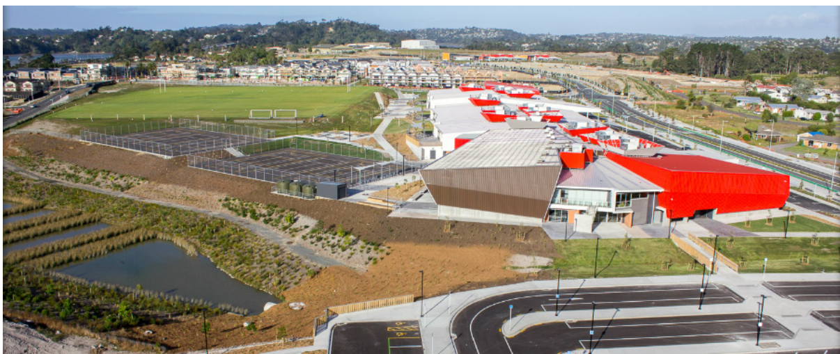
Figure 9: New Hobsonville Point Secondary School
