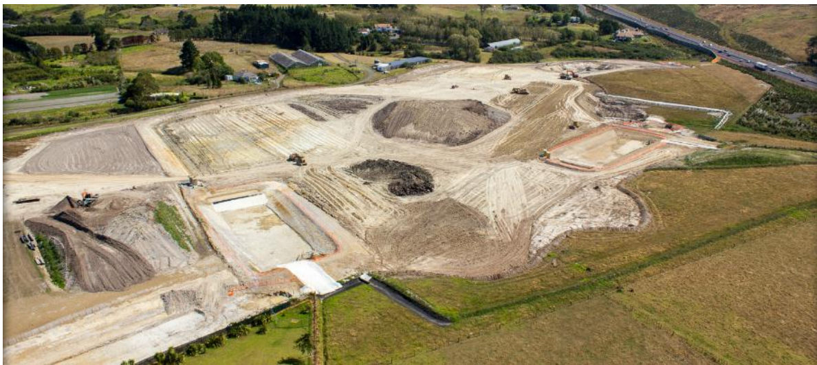
Figure 6: Neil Developments' site looking north to SH 18
