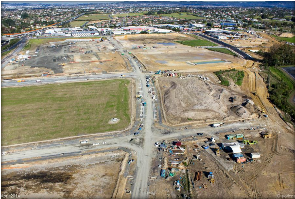
Figure 3: Westgate town centre site looking south to existing shopping centre
