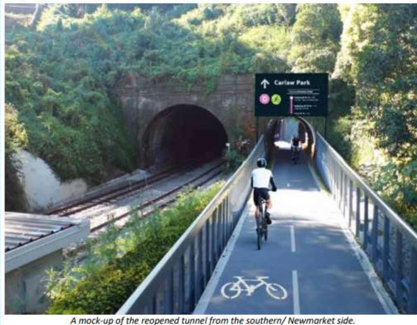
A mock-up of the reopened tunnel from the southern/ Newmarket side.
