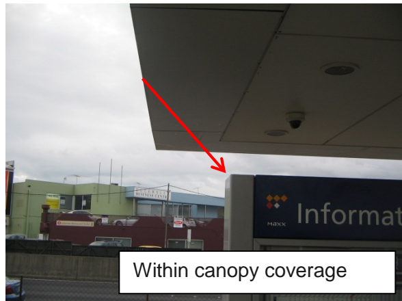
1.2m minimum from top of item to roof edge or at least 0.5m in from roof edge.
