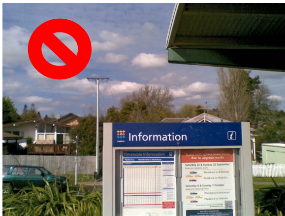
Placing items beneath rungs designed to aid roof access or running directly under the roof edge should be avoided
