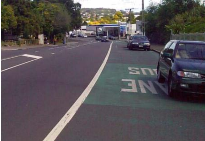
Figure 59: Part time wide shared bus / cycle lane, Auckland
