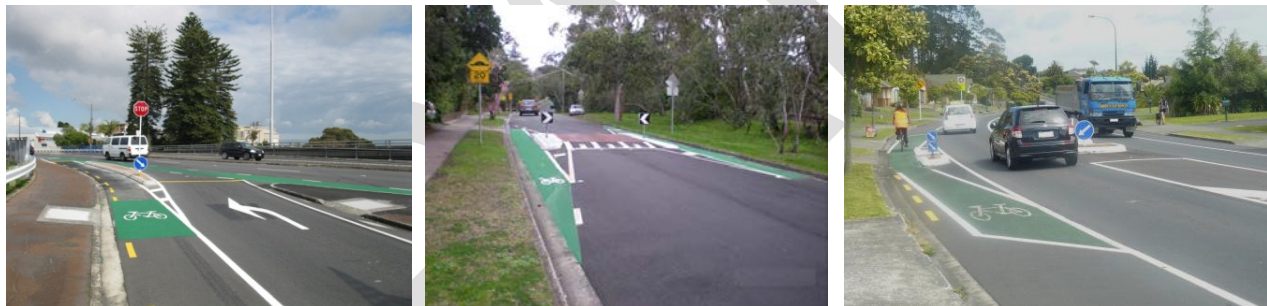
Figure 80: Examples of cycle bypass of speed hump (left, source: Austroad) and cycle bypass at kerb build outs Ian McKinnon Drive Akl (middle), Summerland Drive Akl (right)
