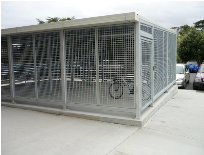
Figure 99: Cycle Parking Cage - Middlemore Hospital (K Hancock)
