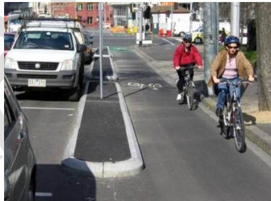
Figure 51: Protected (island) cycle lane, Melbourne
