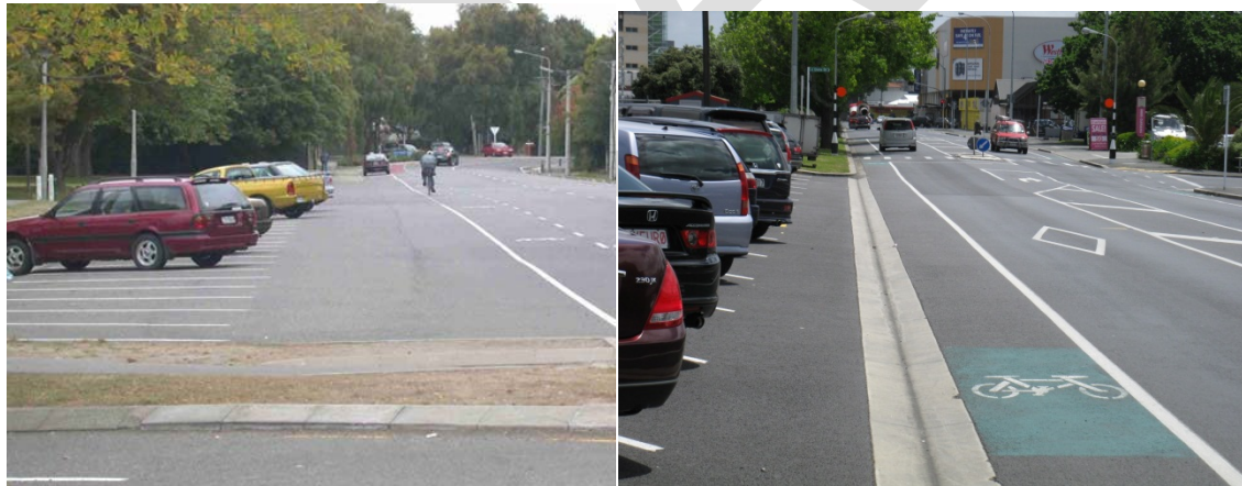
Figure 45: Cycle lane next to angle parking (Christchurch left, Railside Ave, Akl right)
