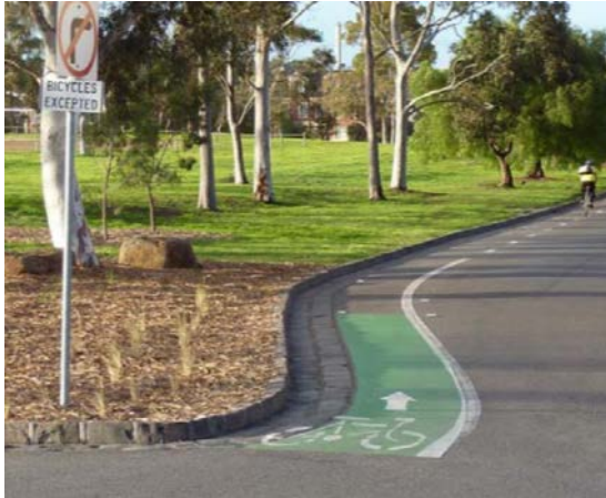
Figure 55: Contra-flow lane on left kerb (one way general traffic approaching viewpoint)
