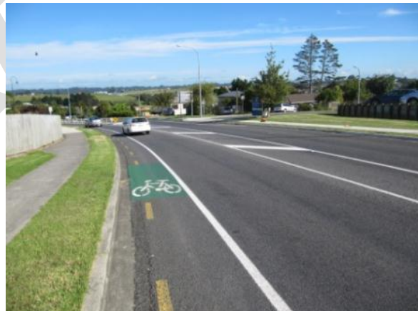
Figure 41: Cycle lane with colour highlight, white cycle logo and "no stopping" lines, Auckland
