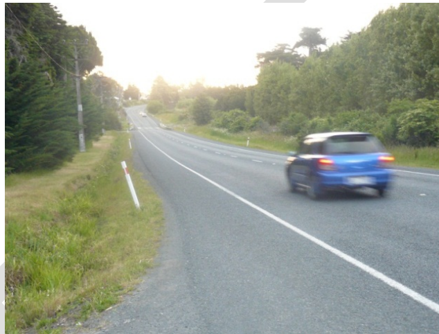
Figure 58: Sealed shoulder, SH16, Akl
