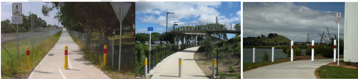
Figure 76: Examples of bollards on shared path from left to right: Austroads (2009m) SH 20 cycleway near Ketih Hay Park (Akl), Waikaraka cycleway (Akl)
