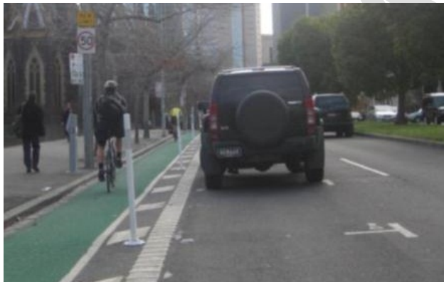
Figure 50: Protected cycle lane (buffer, rumble strip and bollards) with parking between footpath and clearway, Melbourne
