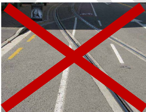
Figure 67: Cycle lane across tram track at oblique angle
