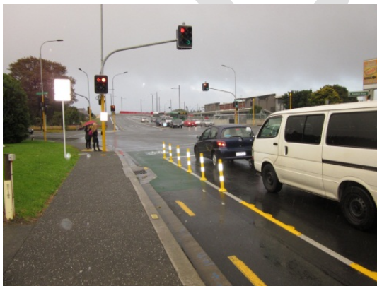
Figure 43: Rubber kerb used in combination with bendable bollards (Auckland, Clark Street, New Lynn)
