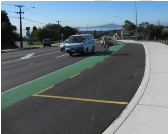
Figure 40: Cycle lane with colour at bus stop layby, North Shore
