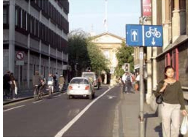
Figure 56: Contra-flow lane on right kerb with standard cycle lane on left of one-way general traffic lane, UK
