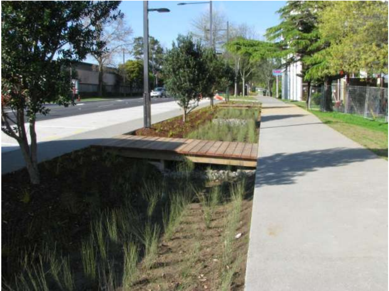
An example of water sensitive design to treatment of stormwater in a street.
