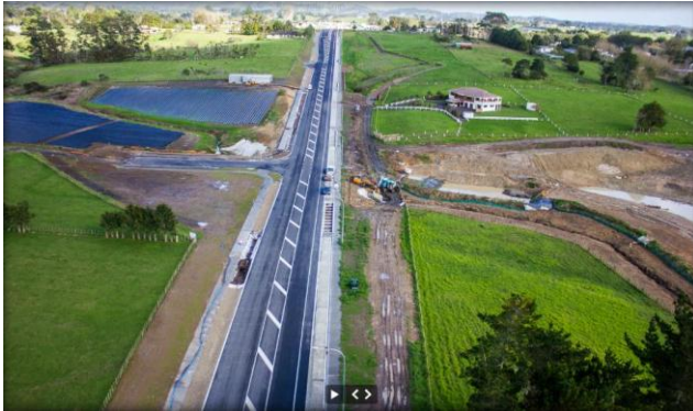
Figure 5: Northside Drive looking west
