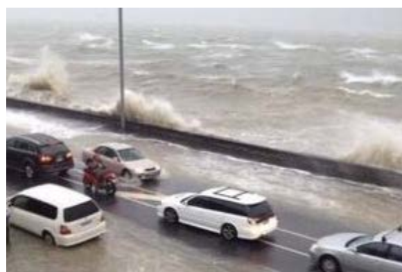
Figure 3-9: Waves overtop the Tāmaki Drive seawall during Cyclone Ita in 2014
