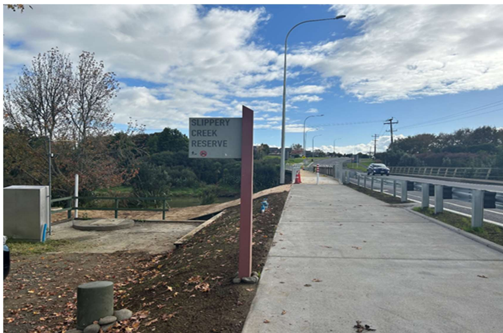
Caption: Otūwairoa Bridge – New Clip-on Footbridge
