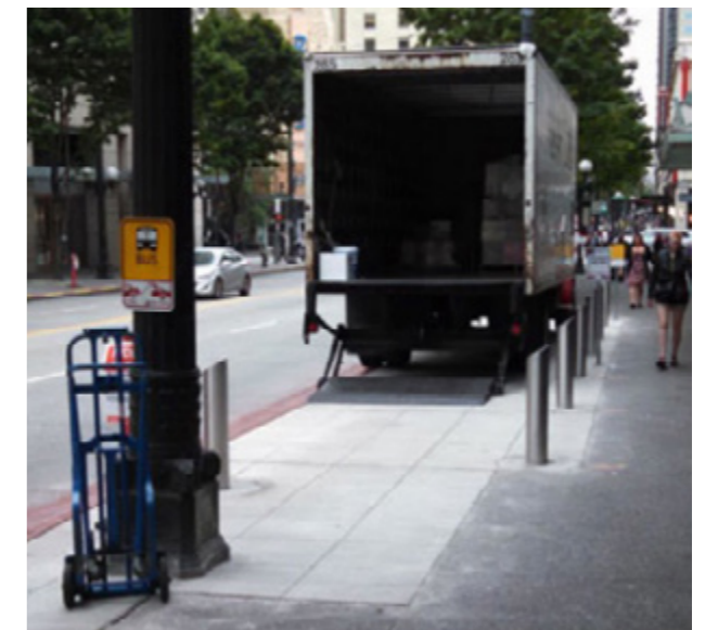
Raised loading zone in Seattle. (Source: Seattle Department of Transportation)
