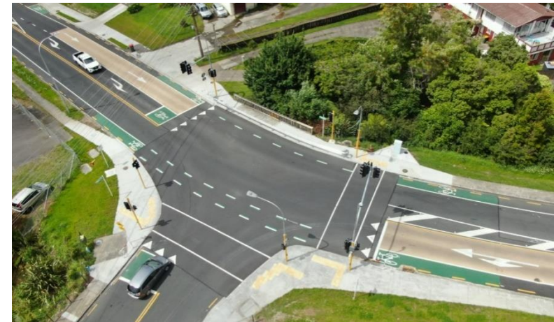
Caption: The new signalised intersection at Triangle Road and Makora Road
