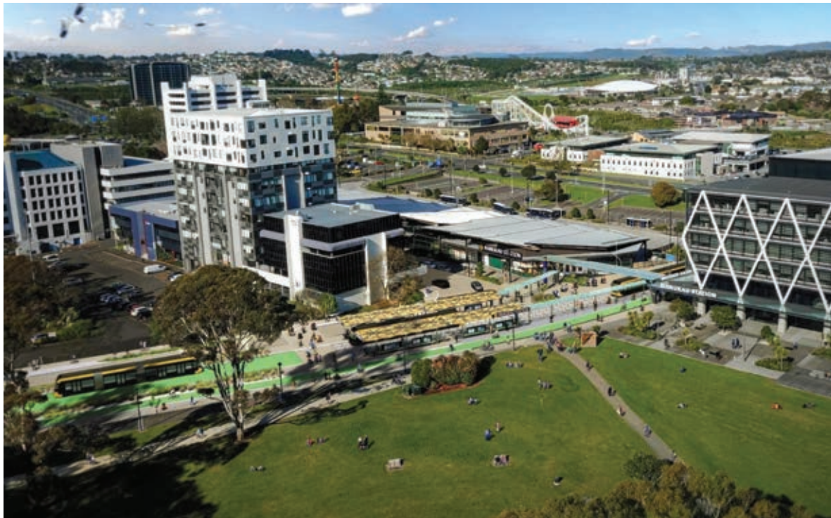
Figure 15-4: A2B rapid transit at Manukau station
