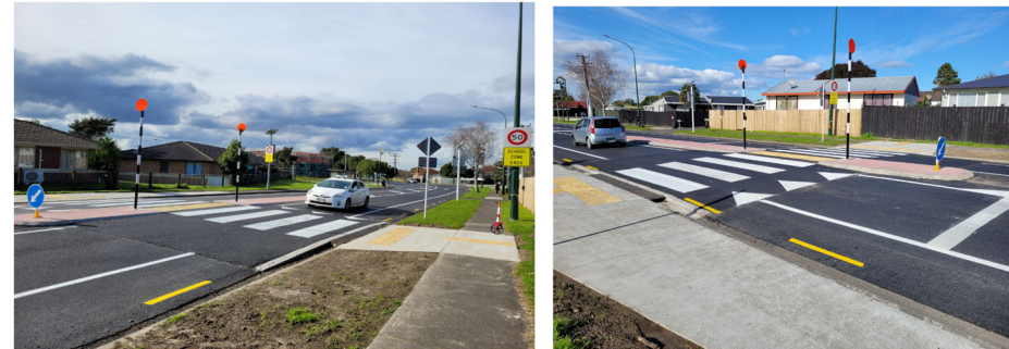
After photos of the new raised zebra crossings on Swanson Road
