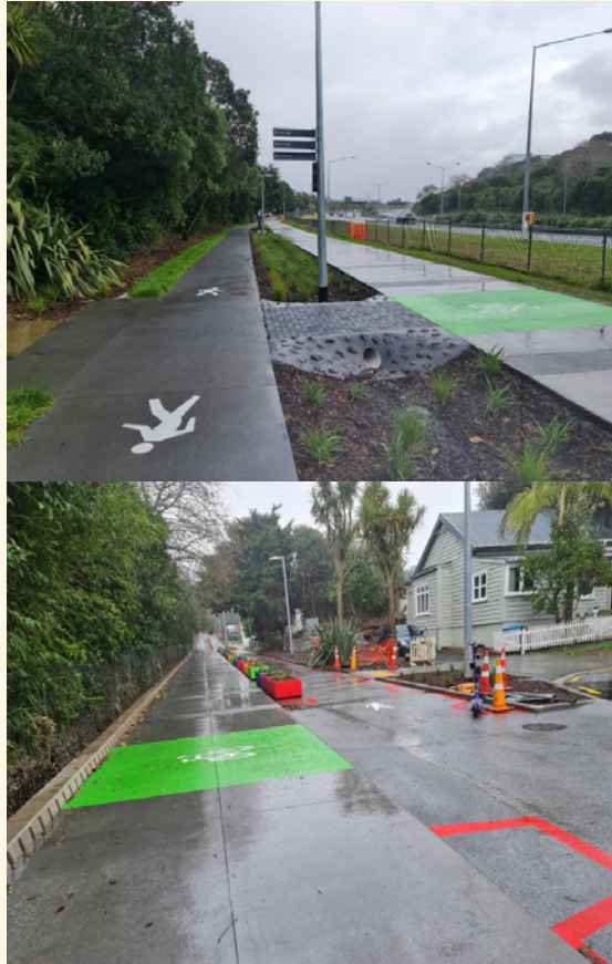
The upgraded North-western Dual Path
