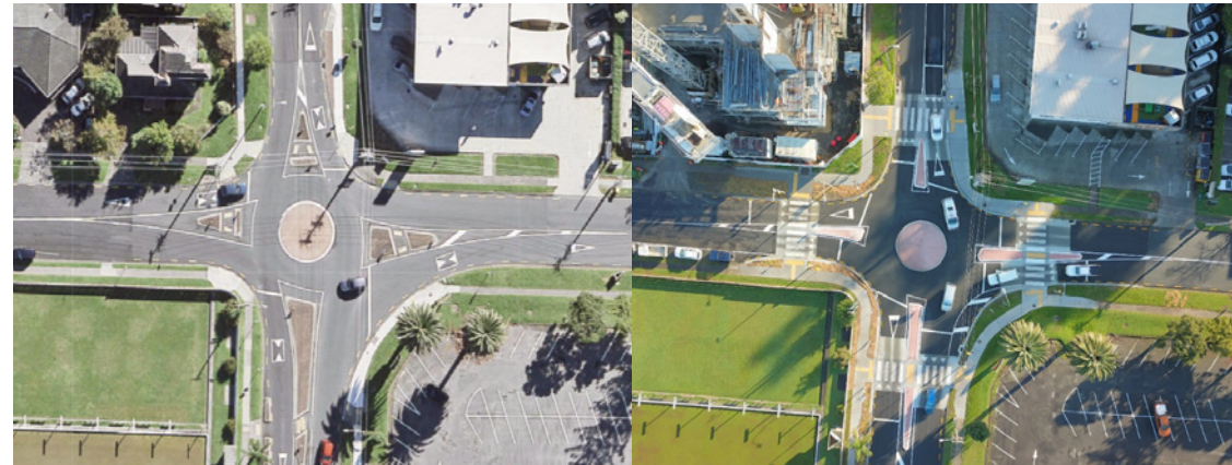
Before and after photos of the Bute Road/Beach Road roundabout improvement project
