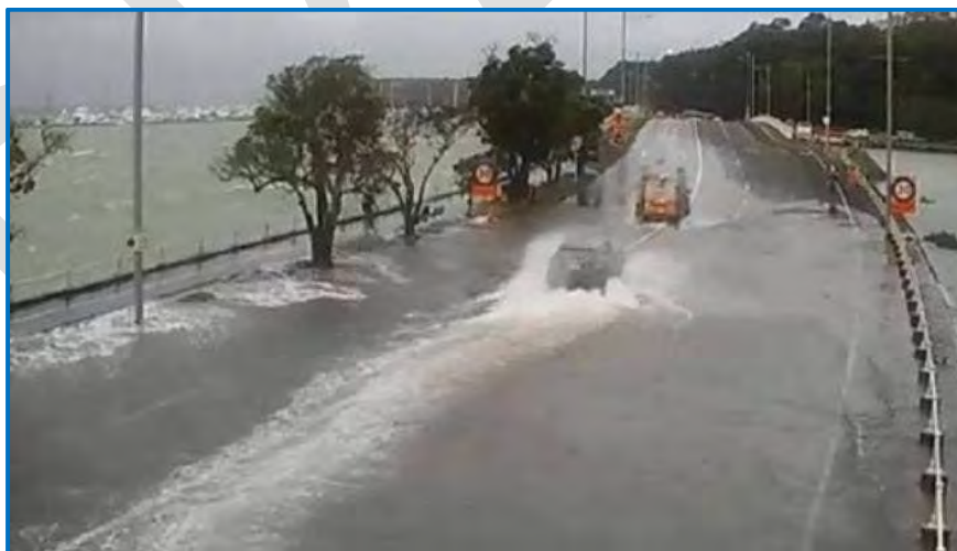
Figure 47 - Flooding on Tamaki Drive in 2018
