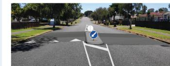
Swedish-style speed tables are a raised table with only one sharp ramp, which produces a smoother ride for buses. Compared to the normal speed table that has two sharp ramps.
