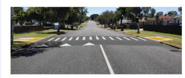
Where pedestrian numbers justify them, zebra crossings will be installed on speed tables. A speed table is a raised section of the road with ramps on each side and a flat surface on top. The white arrows indicate the raised surface and direction of the incline.
