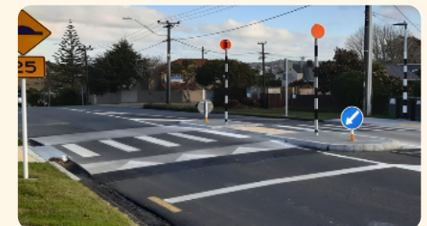
New pedestrian crossings installed on Sunnynook Road, Sunnynook
