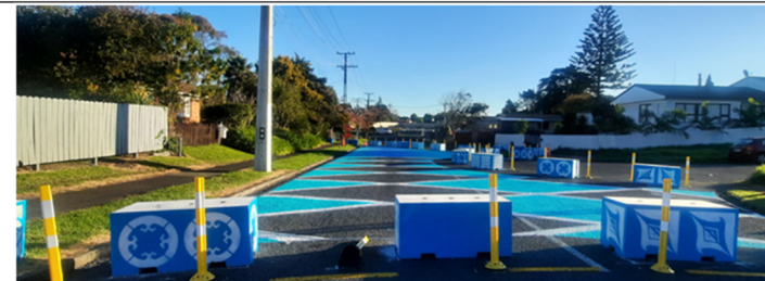
Papatoetoe West Low Traffic Neighbourhood, led by Ōtara-Papatoetoe Local Board seeks to address high speeds and extraneous traffic in the area and encourage uptake of active modes. The pilot includes modal filters to manage speeds and traffic, restricting where vehicular traffic can travel. Modal filters have received mixed feedback and the local board have decided to modify the layout of both modal filters in response.
