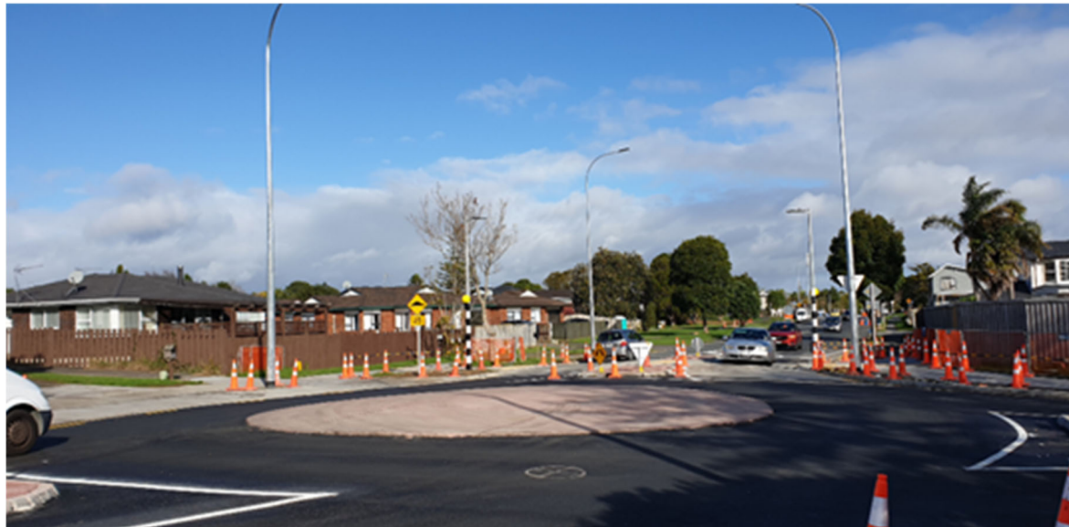
Figure 2 New roundabout constructed at intersection of Bucklands Beach and Sunderland's Roads
