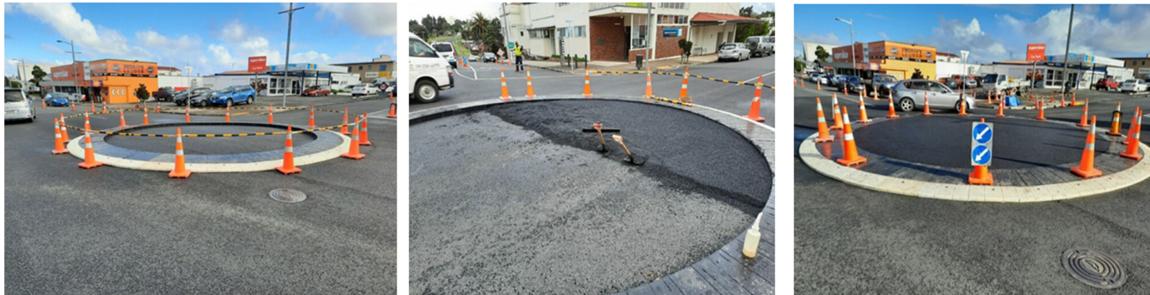
Figure 4 New rubber roundabout installed in Waiuku
