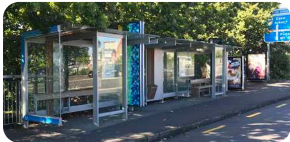
GOOD QUALITY ON-STREET BUS FACILITY AT SYMONDS STREET
