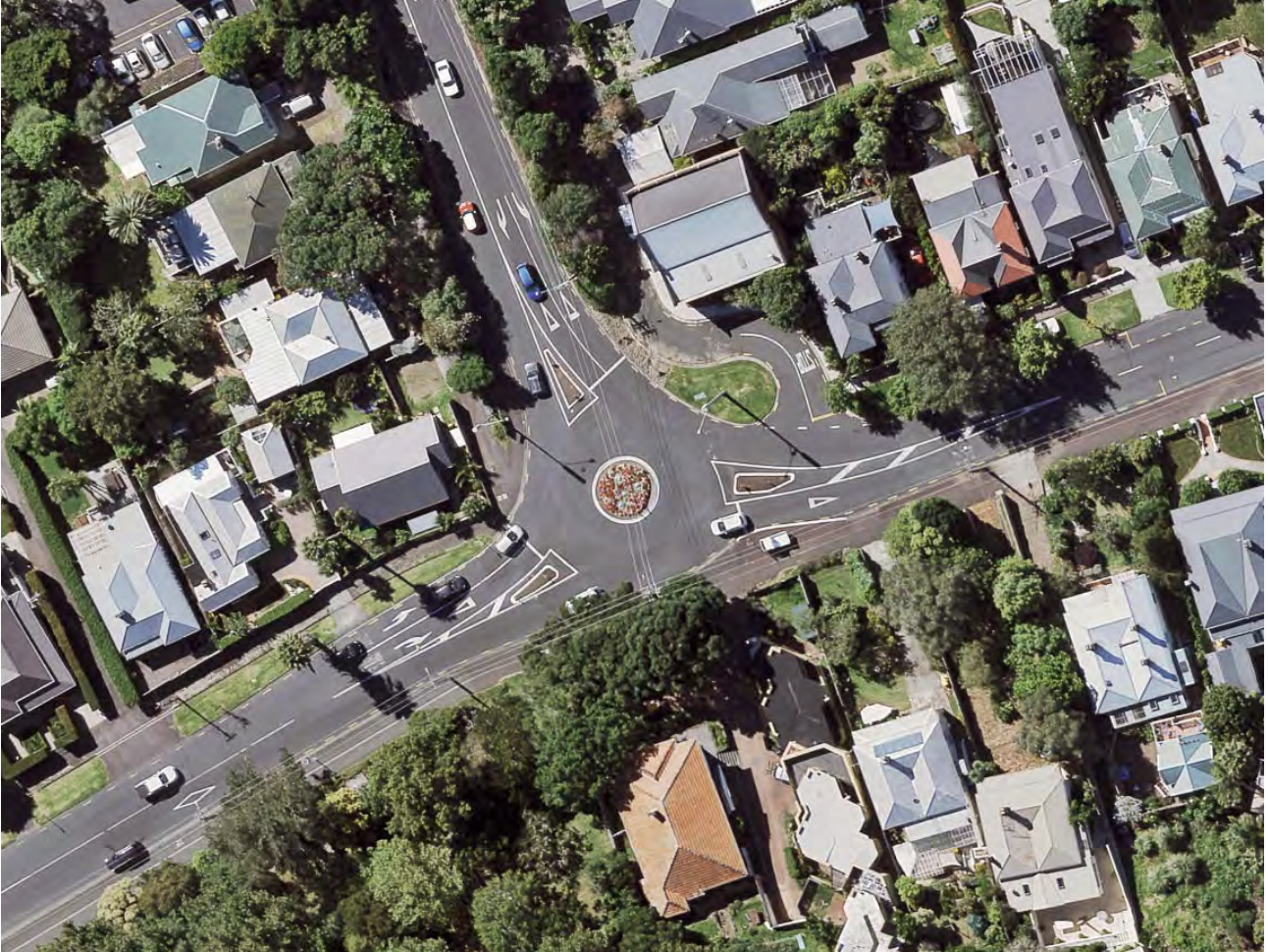
Figure 7-51 Lake Road / Albert Road Roundabout – Existing Layout
