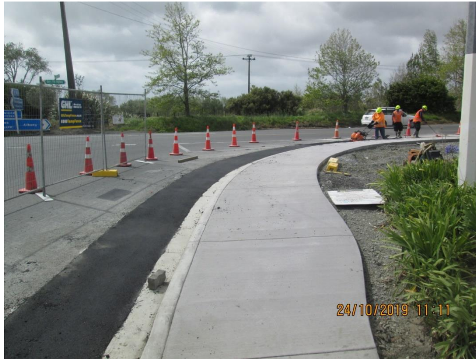
Photograph of left turn slip removal at Kahikatea Flat Road
