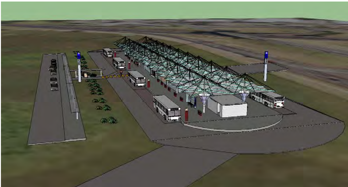
Figure 24: Intermediate Interchange with a central island
