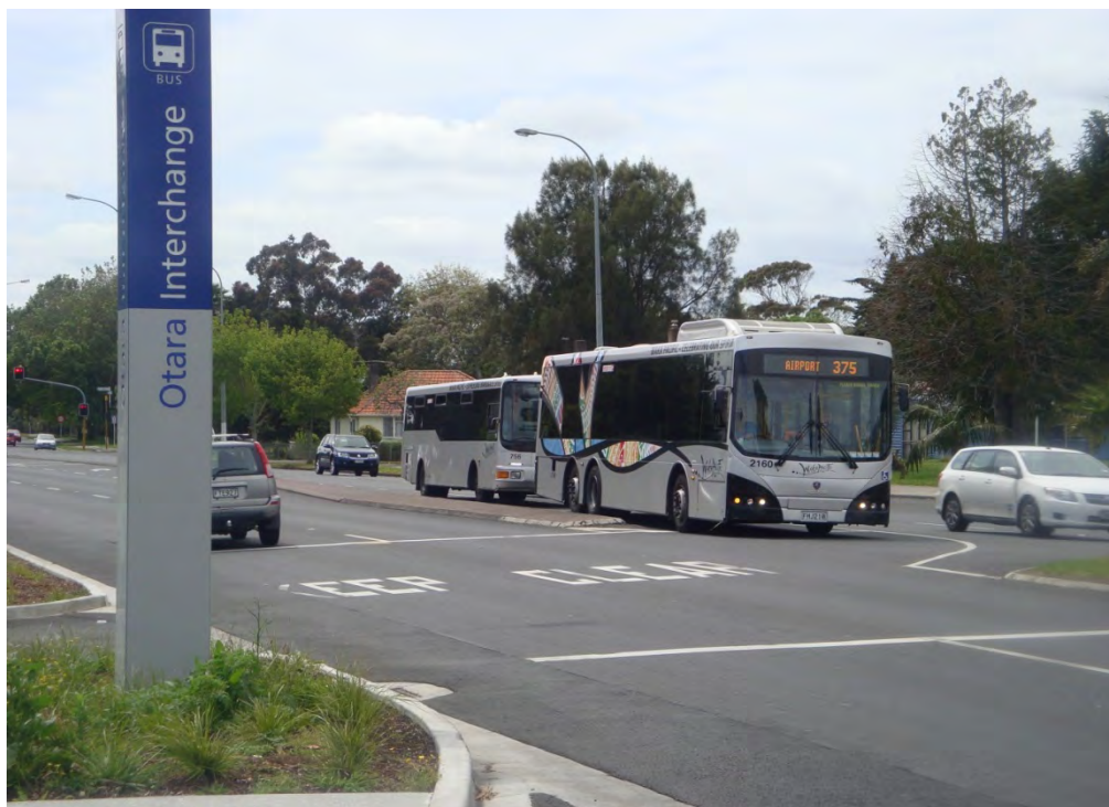
Figure 1: Eastern entrance to Otago Interchange
