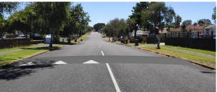
A speed hump is a short rounded raised section of the road. The white arrows indicate the raised surface and direction of incline.
