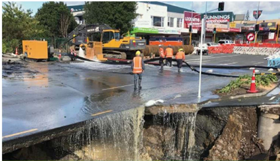
Figure 6-5: Closure of Great North Road, New Lynn
