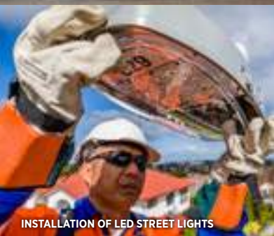
INSTALLATION OF LED STREET LIGHTS
