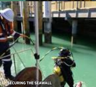
SECURING THE SEAWALL
