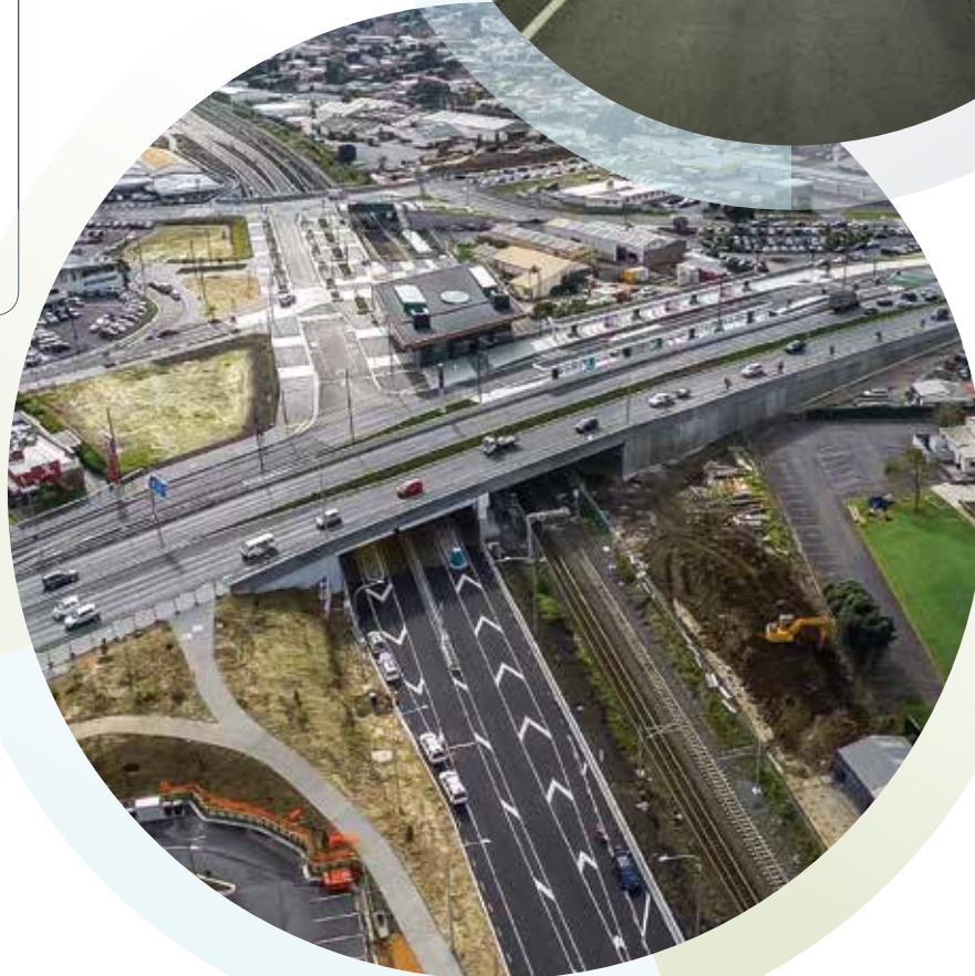
Te Horeta Road tunnel.
