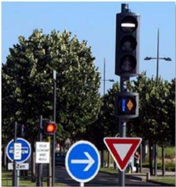
BRT signal aspect
