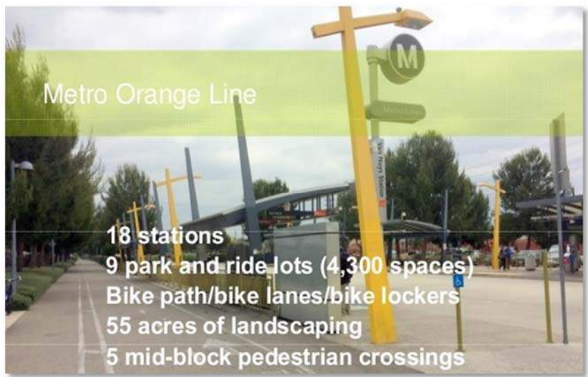
The Orange Line in LA County, USA
