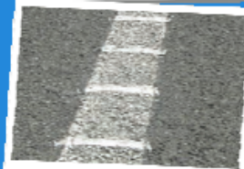
A rumble strip
