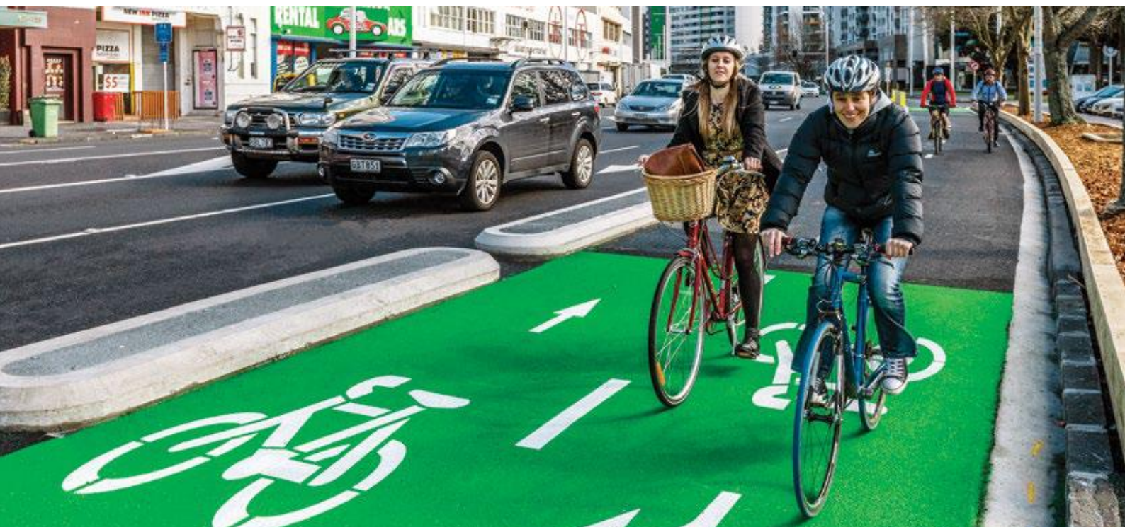
Auckland's first on-road separated cycleway at Beach Rd linking to the Grafton Gully and North Western cycleways
