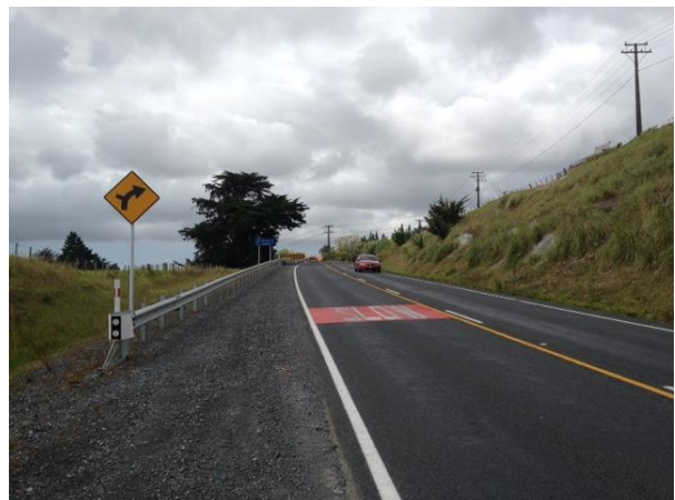
After photo – Intersection warning sign, Slow pad and guardrail installation
